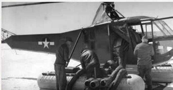
A portable heating unit had to be flown in to warm the engine when the Sikorsky would not start one cold morning at the weather station/radio-range site on Lake Morhiban. USAAF Photo
